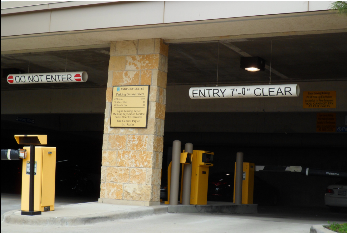
FIGURE 2. Parking Garage. The vertical clearance for this parking garage is posted at 7'0" and is required to be a minimum of 8'2".
