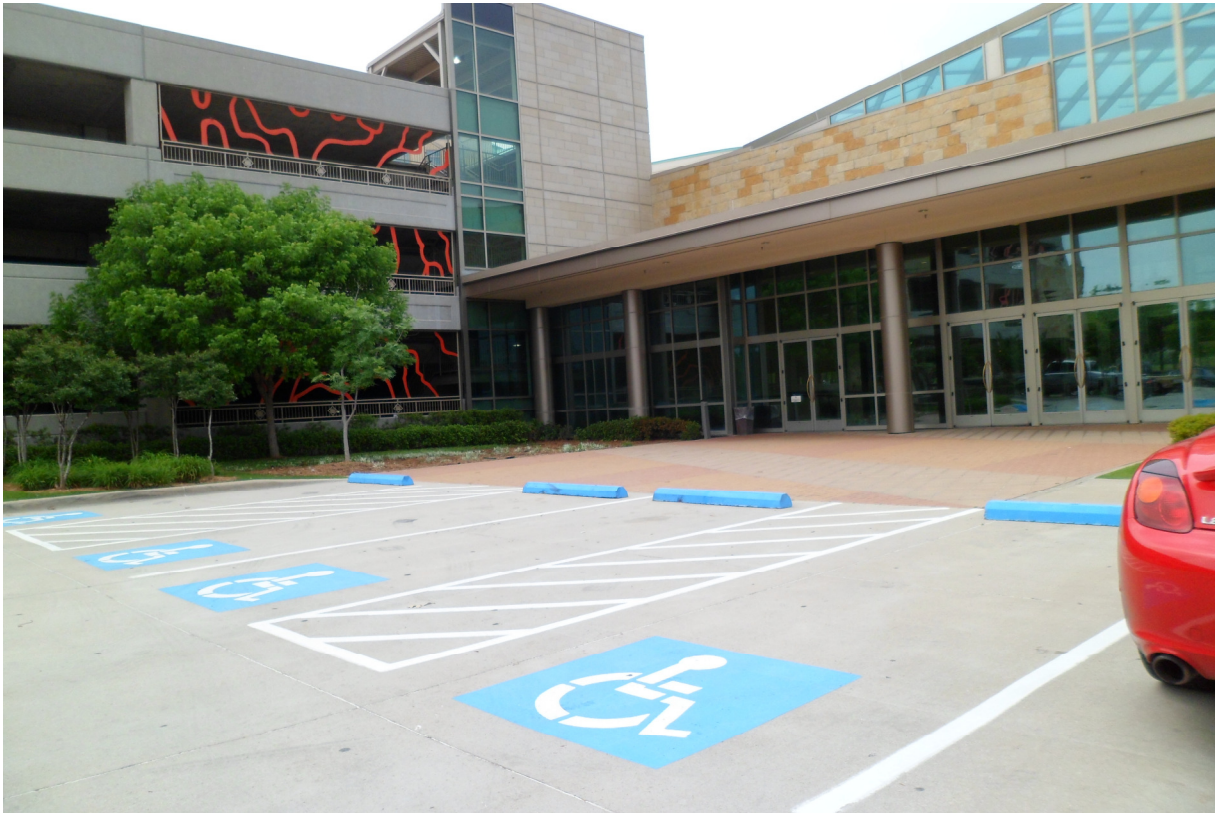
FIGURE 1. Parking: This lot is required to have 5 spaces and only has 4. None of them have the required signage.
