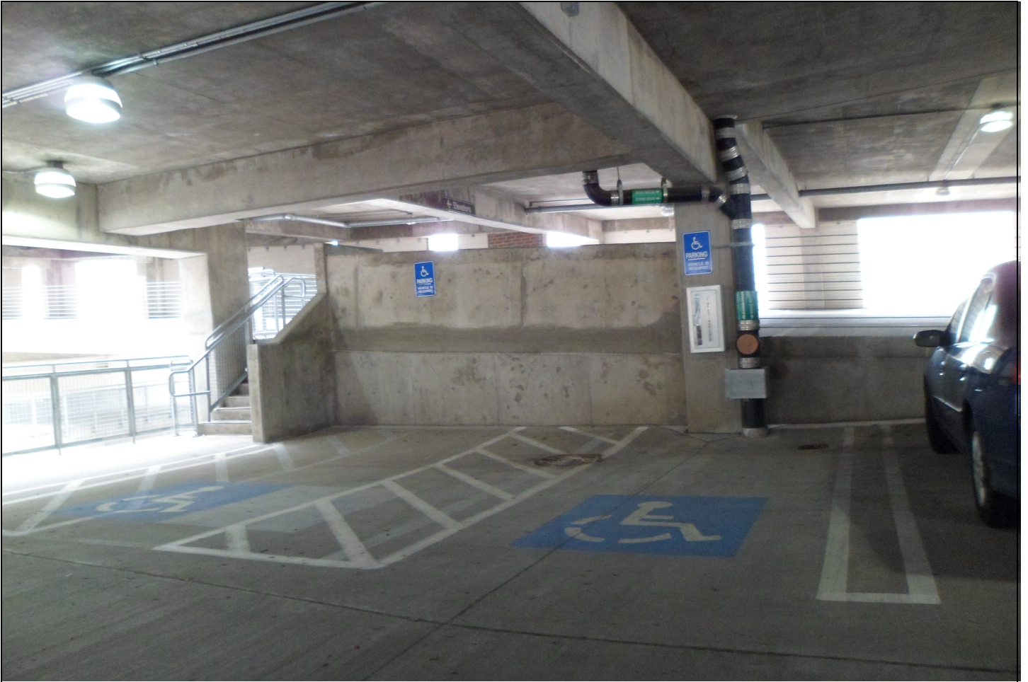
FIGURE 3. Accessible parking spaces - The front of these accessible parking spaces slopes up. The entire accessible parking space and it's associated access aisle are not allowed to have more than a 2% slope.
