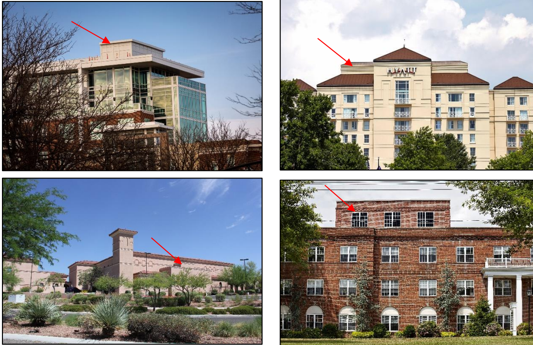
Figure 7.01.1: Examples of Stealth Antenna Rooftop Concealments
