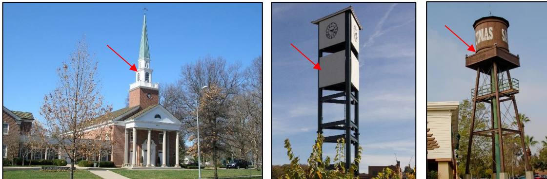
Figure 7.01.2: Examples of Stealth Antenna Steeple and Tower Concealments
