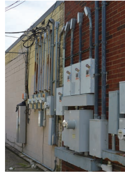
Existing service connections along Downtown Frisco alleys (Source: Garver)
