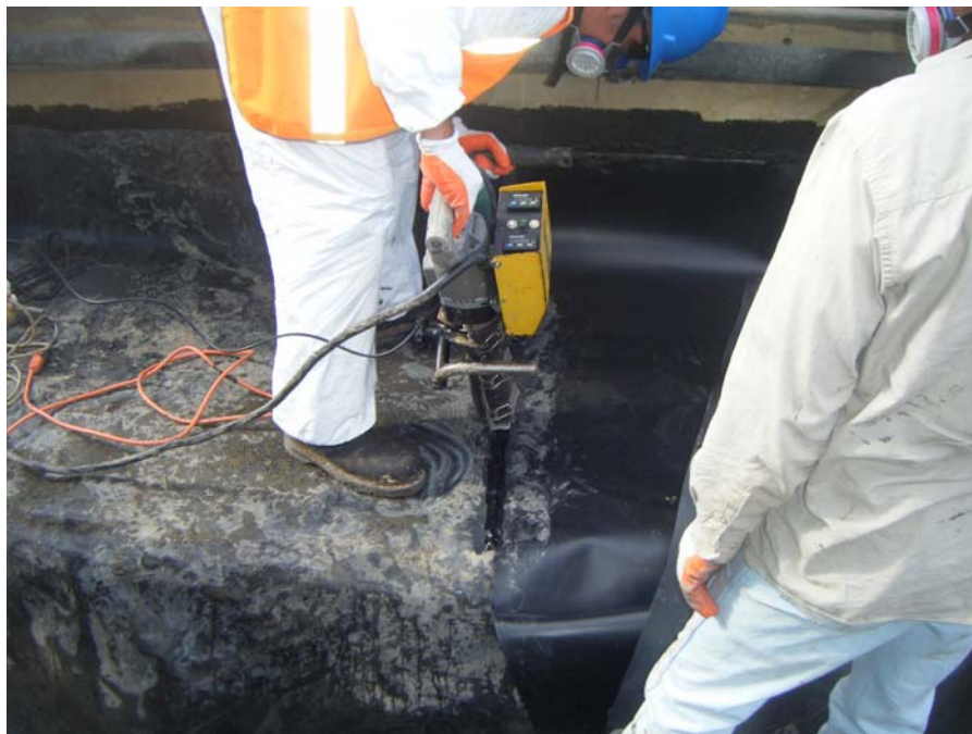
Photo 17: Heat weld of HDPE liner against wall.
