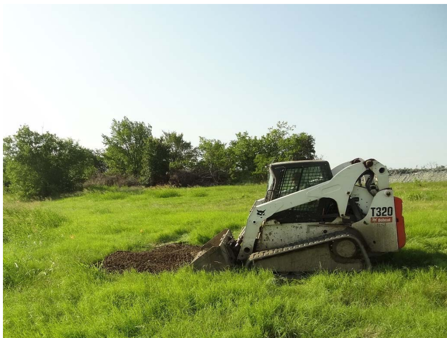
Photo 8: Feathering out clay cap.
