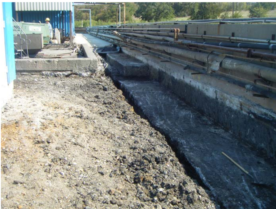
Photo 15: Exposed wall and footing near truck wash.
