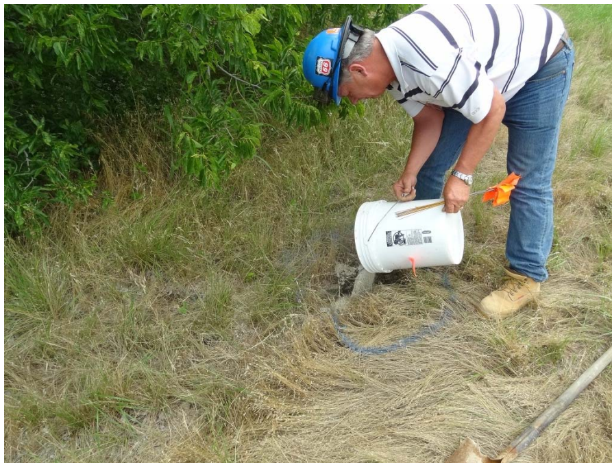
Photo 5: Filling of animal burrow within the SDA with fine grained bentonite chips.
