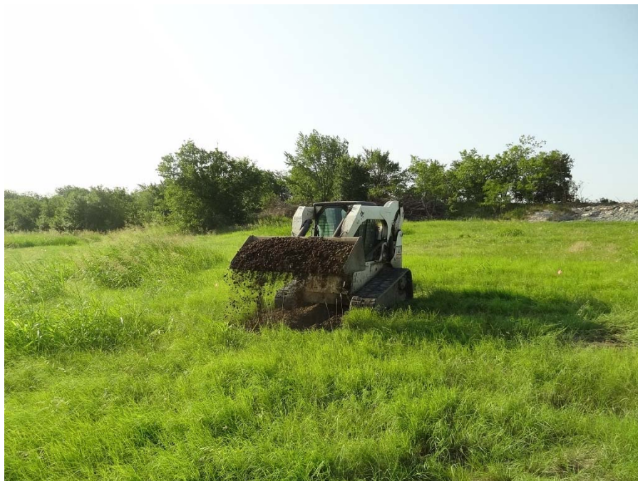
Photo 7: Capping animal burrow (cap-01) along western SDA boundary as viewed to the east.
