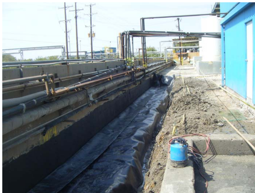
Photo 18: Installed liner prior to drain pipe and anchoring to wall.
