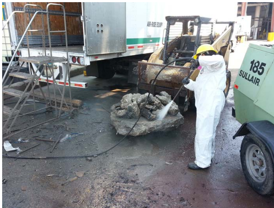
Photo 6: Pressure washing of concrete prior to removal and disposal.
