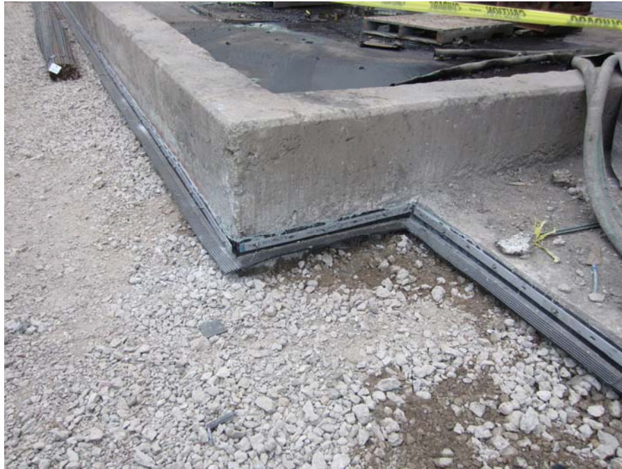
Photo 21: Water stop detail at corner.
