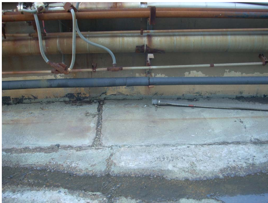
Photo 4: Deteriorated concrete and drainage swale that conveys water to sediment pit.
