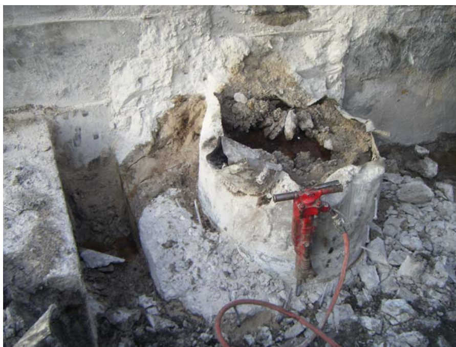
Photo 28: Former sump area, infilled with concrete.
