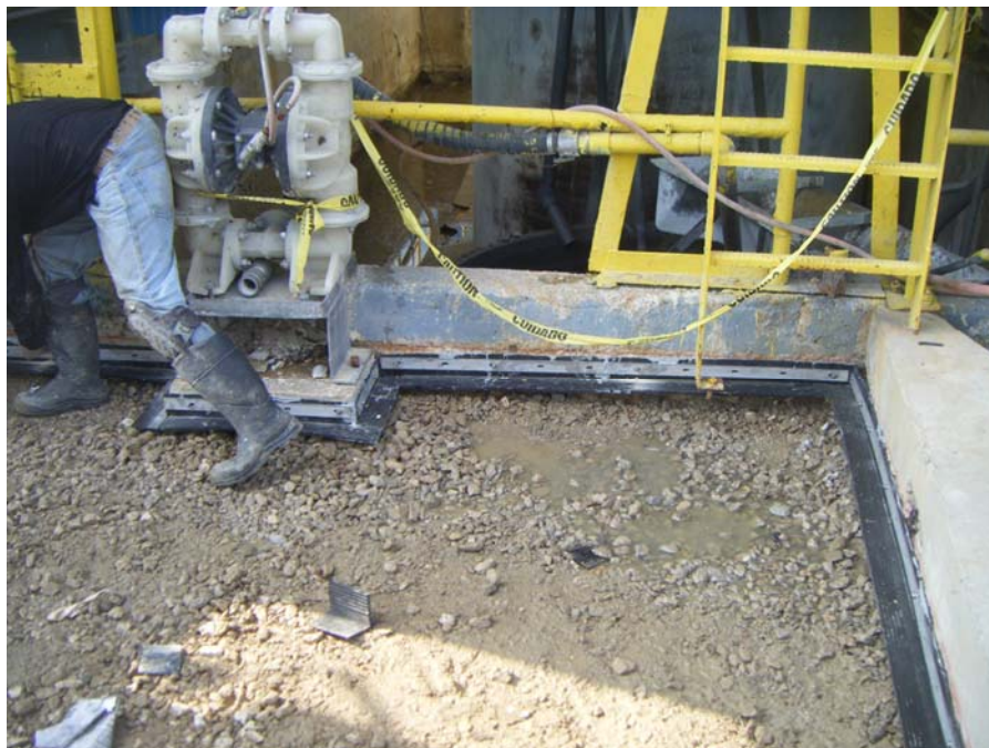
Photo 19: Detail of water stops.
