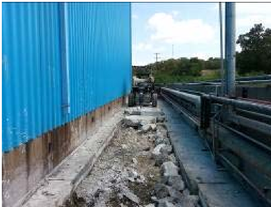
Photo 5: Breaking of concrete in first section, east end of project area..
