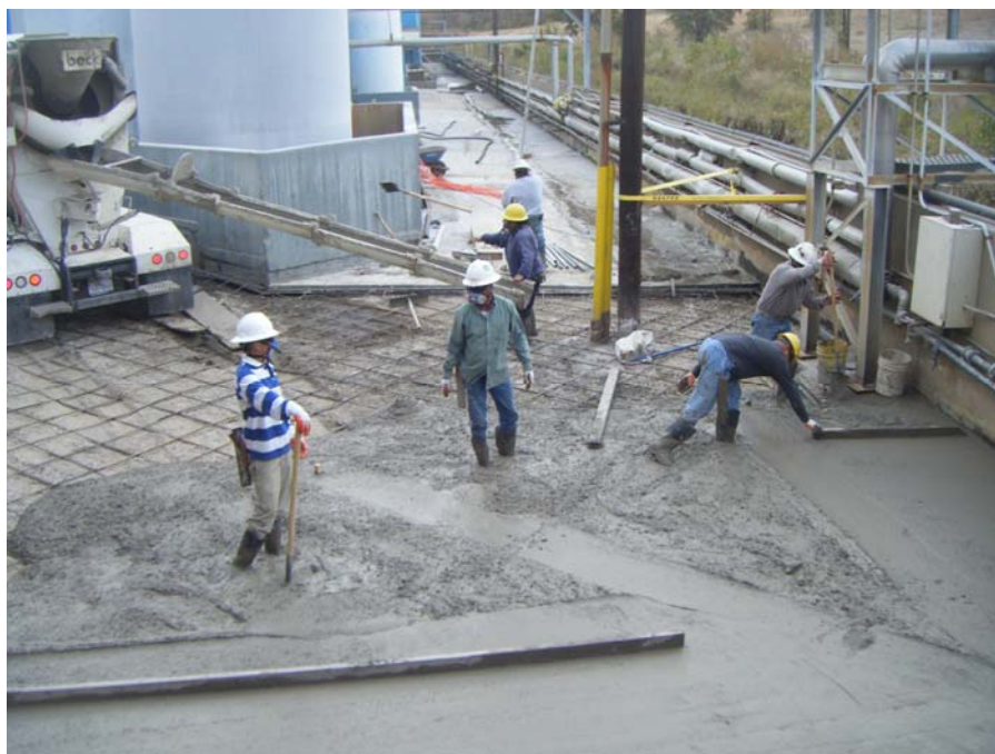
Photo 32: Finishing concrete surfacing at far west end of project.
