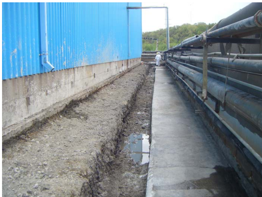
Photo 8: Trench at wall footing prior to installation of drain.
