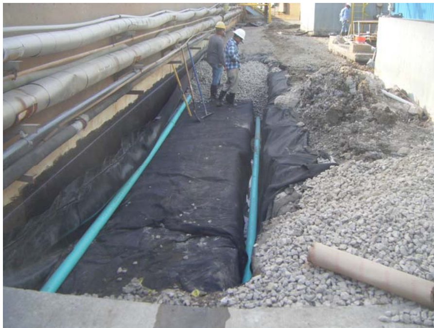
Photo 25: View of stem drain and footing drain installation prior to backfilling.
