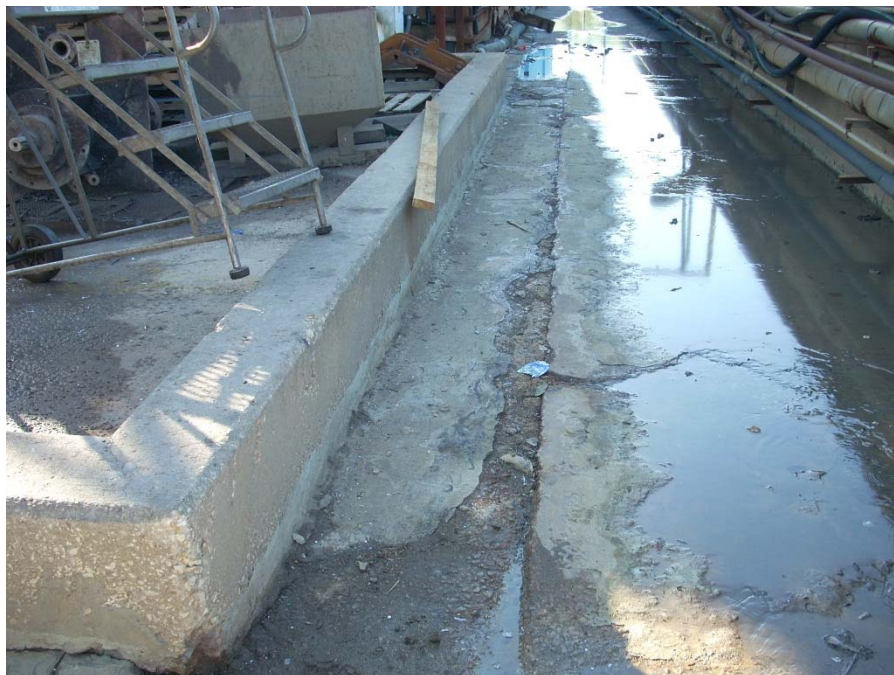
Photo 3: Pre-repair—deteriorated concrete pavement and standing water along retaining wall.
