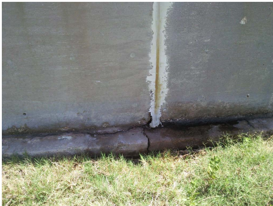
Photo 1: View of area of seepage along exterior face of retaining wall; note staining of caulking and cracks in concrete wall footing.
