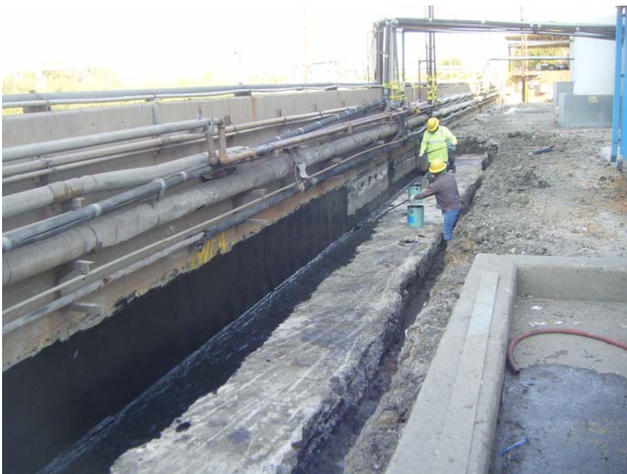
Photo 16: Applying liquid asphaltic membrane to wall stem and footer.
