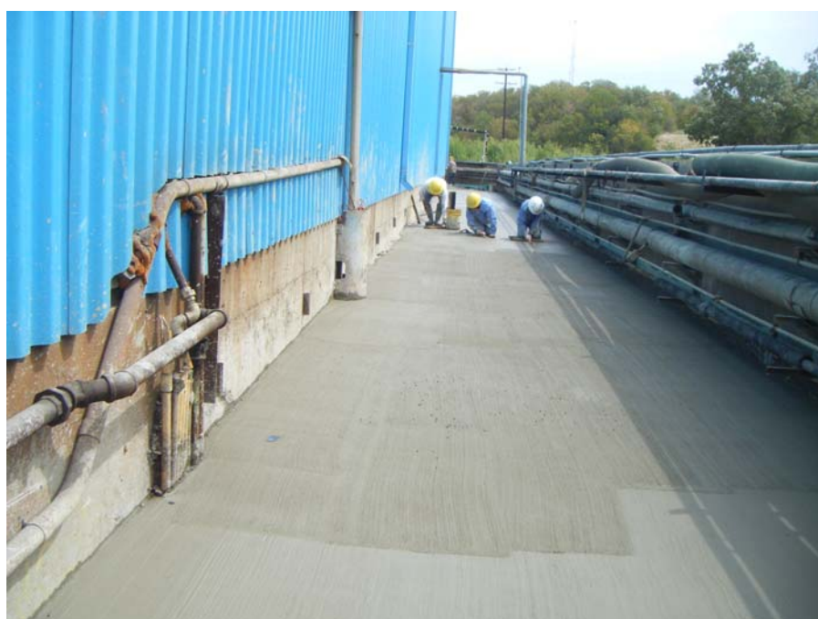
Photo 12: Finishing new concrete paved surface and swale.
