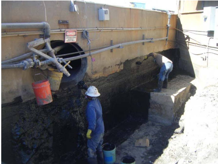
Photo 29: Applying liquid asphaltic membrane at far west end of project.
