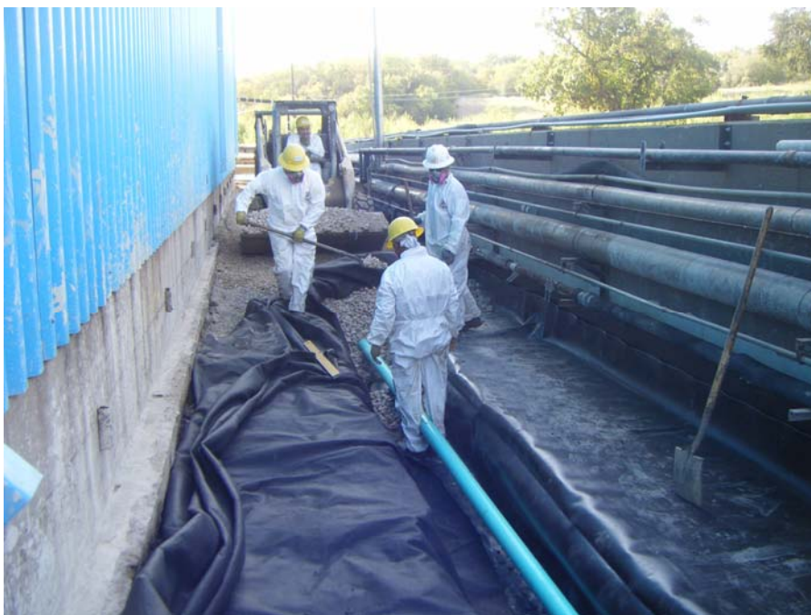
Photo 10: Installing filter fabric for footing drain.
