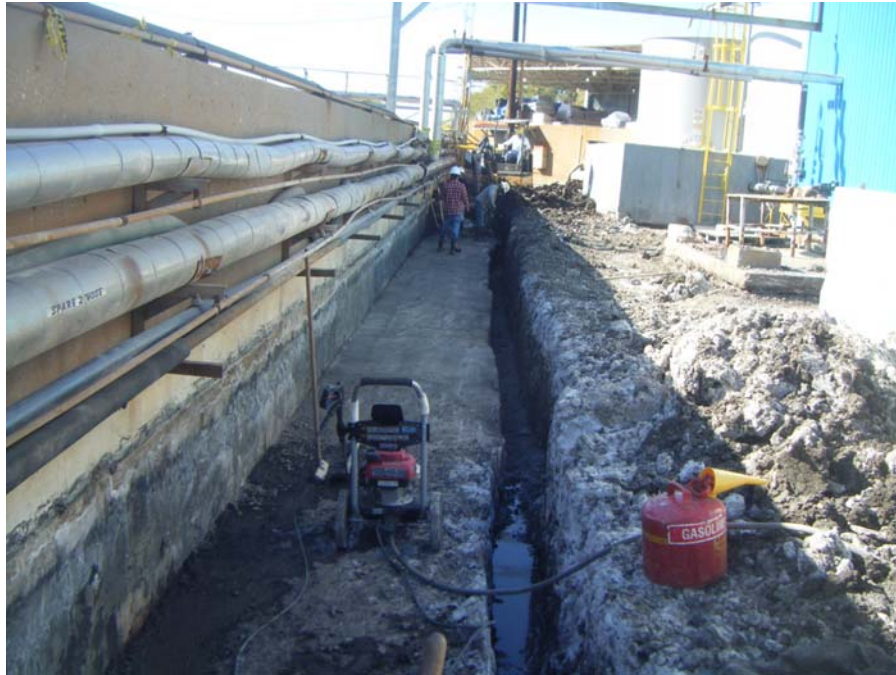
Photo 23: Exposed wall and drain trench prior to membrane and pipe.
