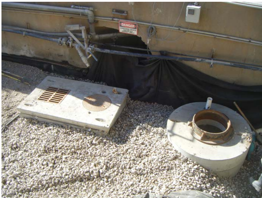
Photo 31: Sump and underdrain manhole after backfilling
