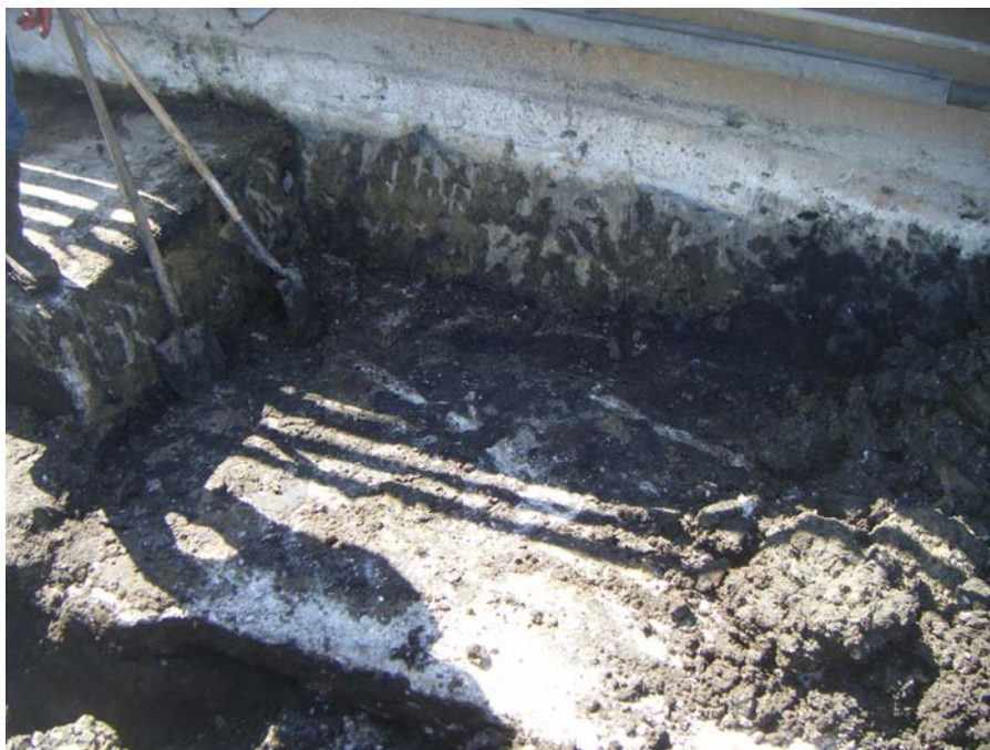
Photo 14: Exposed footing at step-down section.
