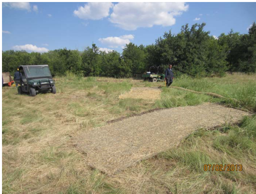
Photo 14: Completed area with erosion mat in place.
