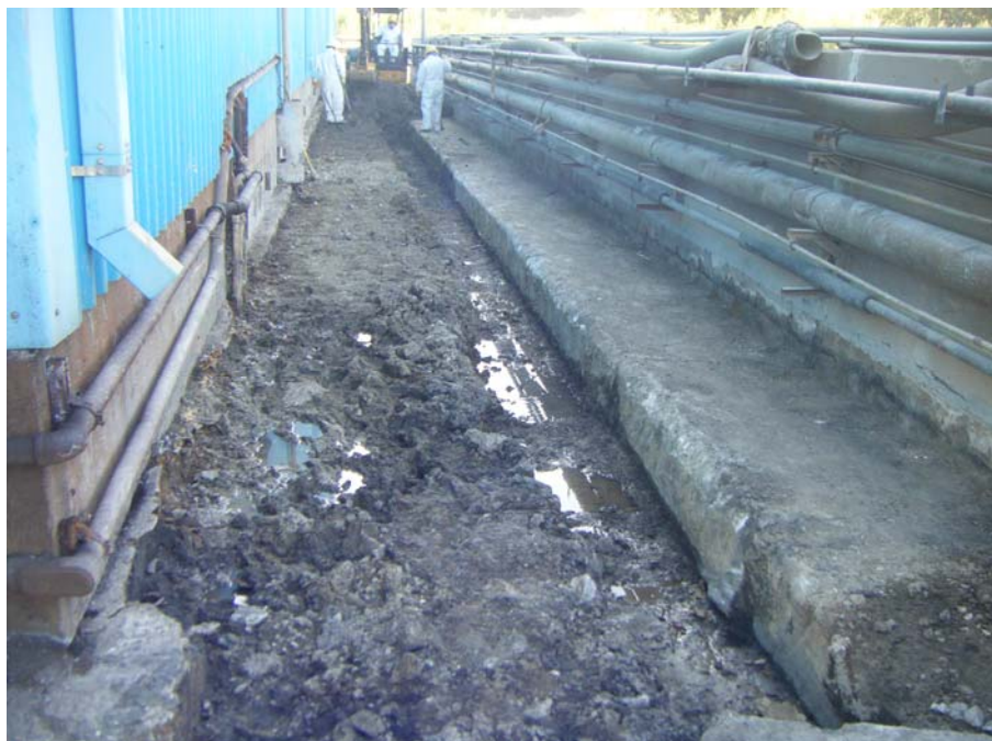
Photo 7: Exposed soil and back of retaining wall footing.
