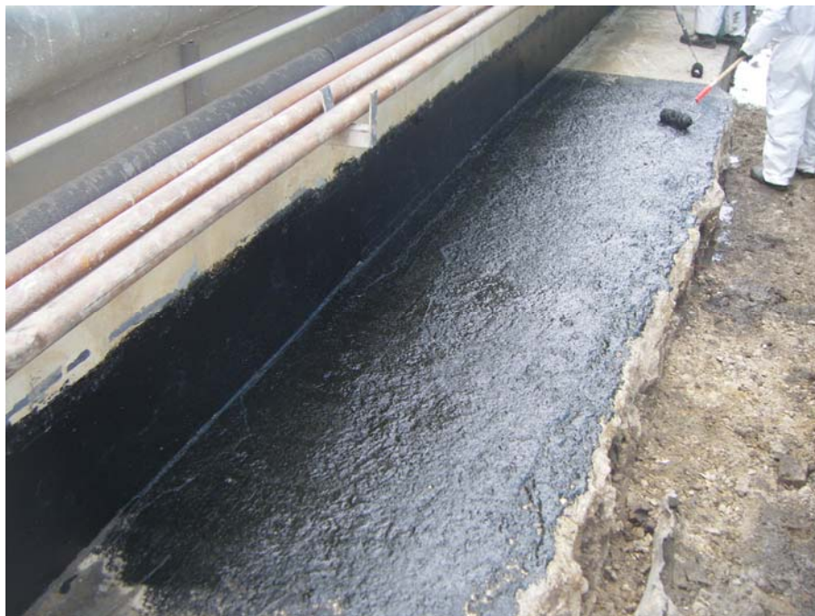
Photo 9: Applying liquid asphaltic membrane to wall and top of footing.
