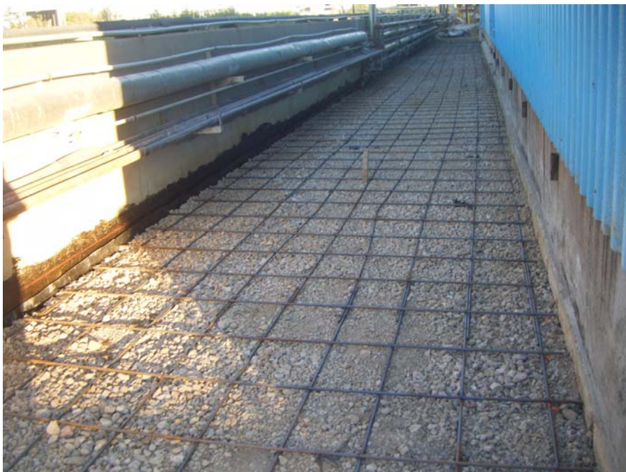
Photo 11: Re-bar installed on flex base awaiting concrete.
