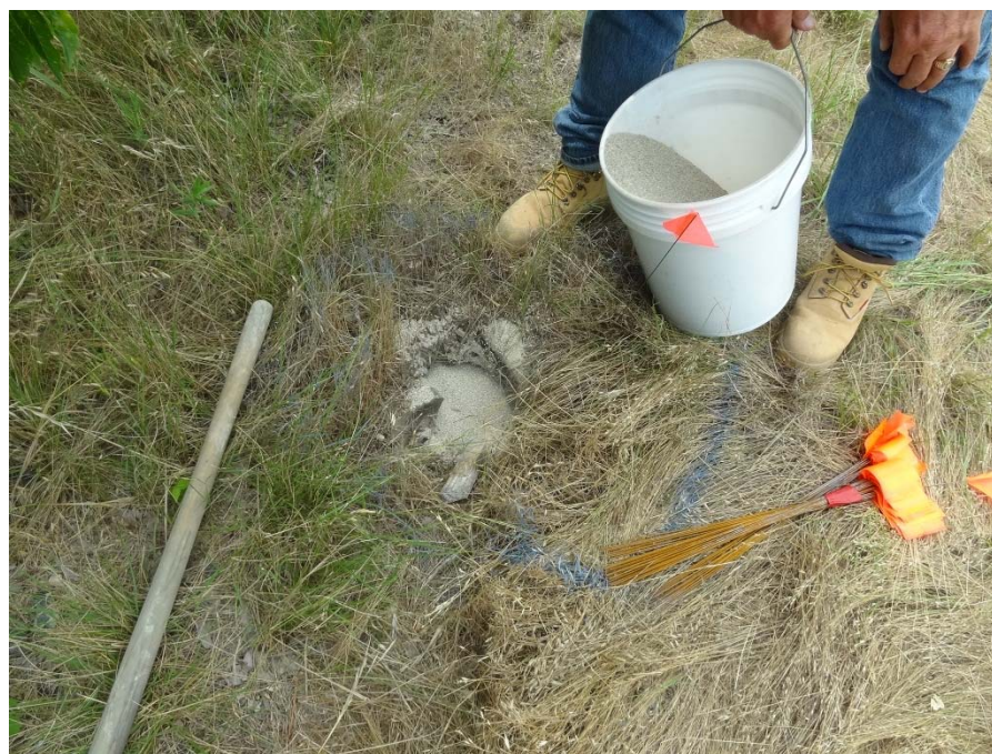
Photo 6: Bentonite filled animal burrow.
