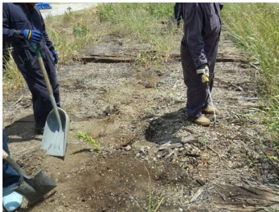
Photo 12: Water misting soil in removal area to eliminate airborne particulates.
