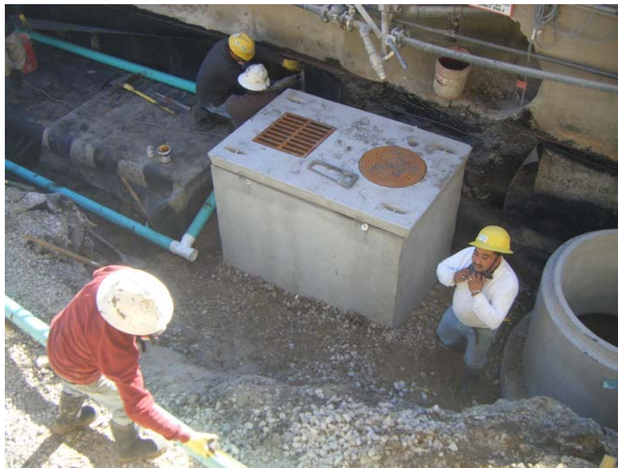
Photo 30: Installation of sump for surface drainage
