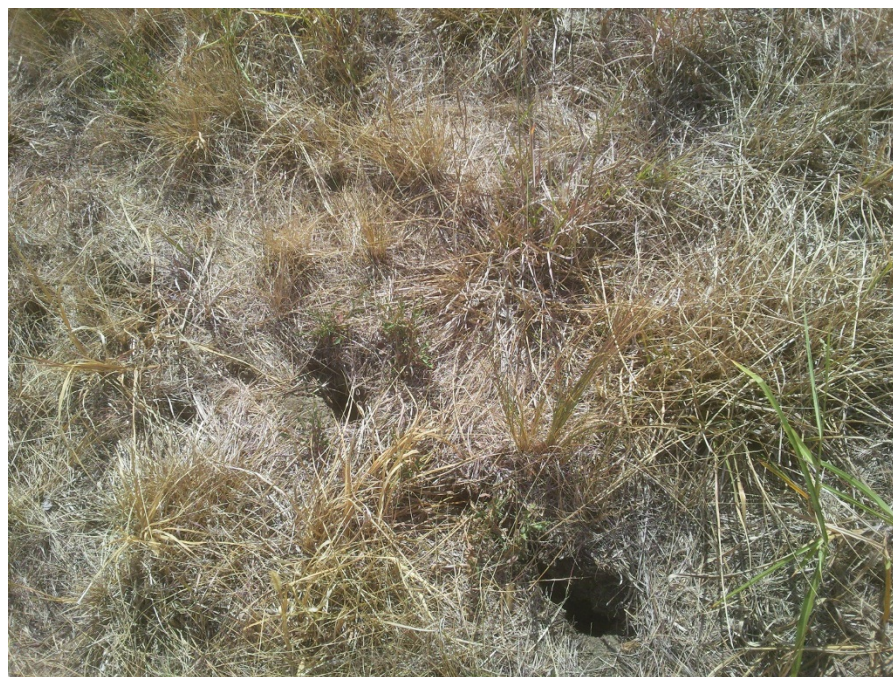
Photo 2: Cracks in SDA cap caused by drought.
