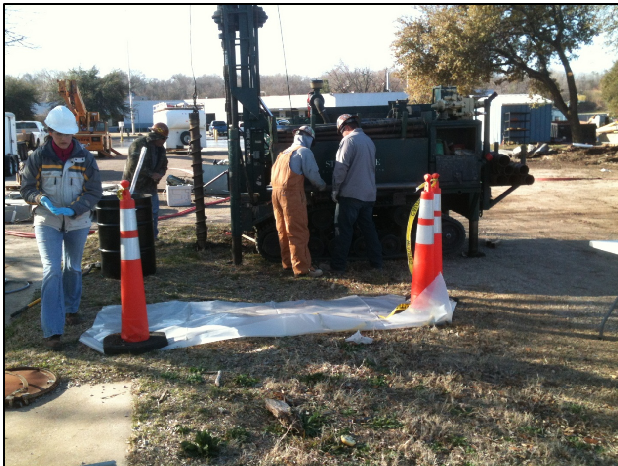
Photo 11 Installation of monitoring well MW-23 on southeast side of Bale Stabilization Area (March 2013).
