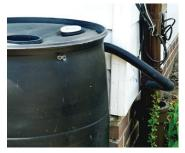
Connecting separate piping to redirect overflow water away from the barrel, plants, and your foundation may be necessary. There are many methods of doing this and the bulk head fitting method may be used again. It is important to note you must protect the barrel from insect and/ or rodent access, so netting should be introduced either at the barrel connection or at the end of the pipe.
