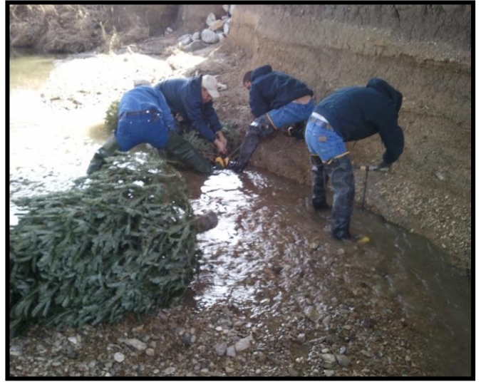
Installation of an evergreen revetment to reduce erosion
